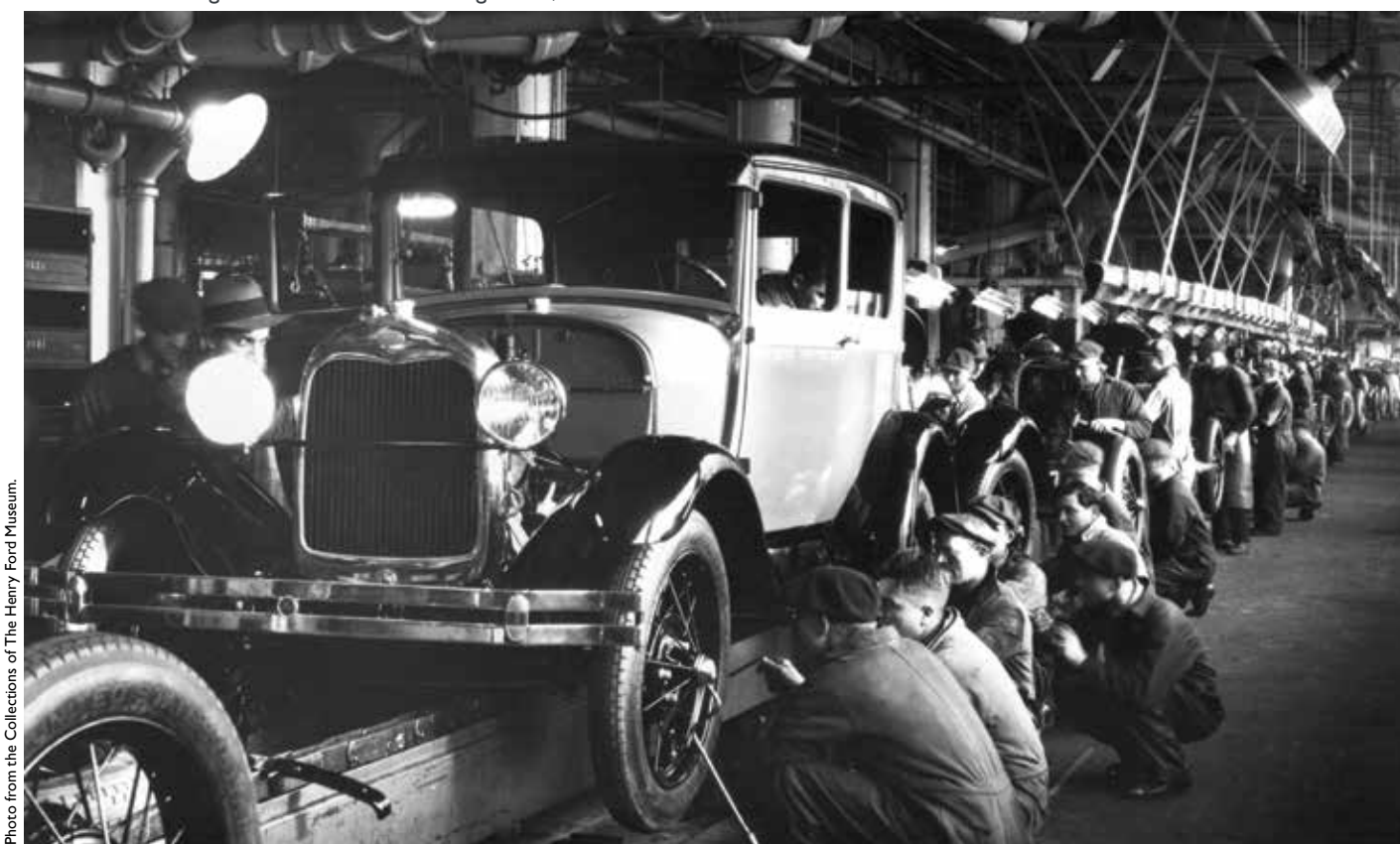
Workers assembling Ford Model As at the Rouge Plant, 1928.
