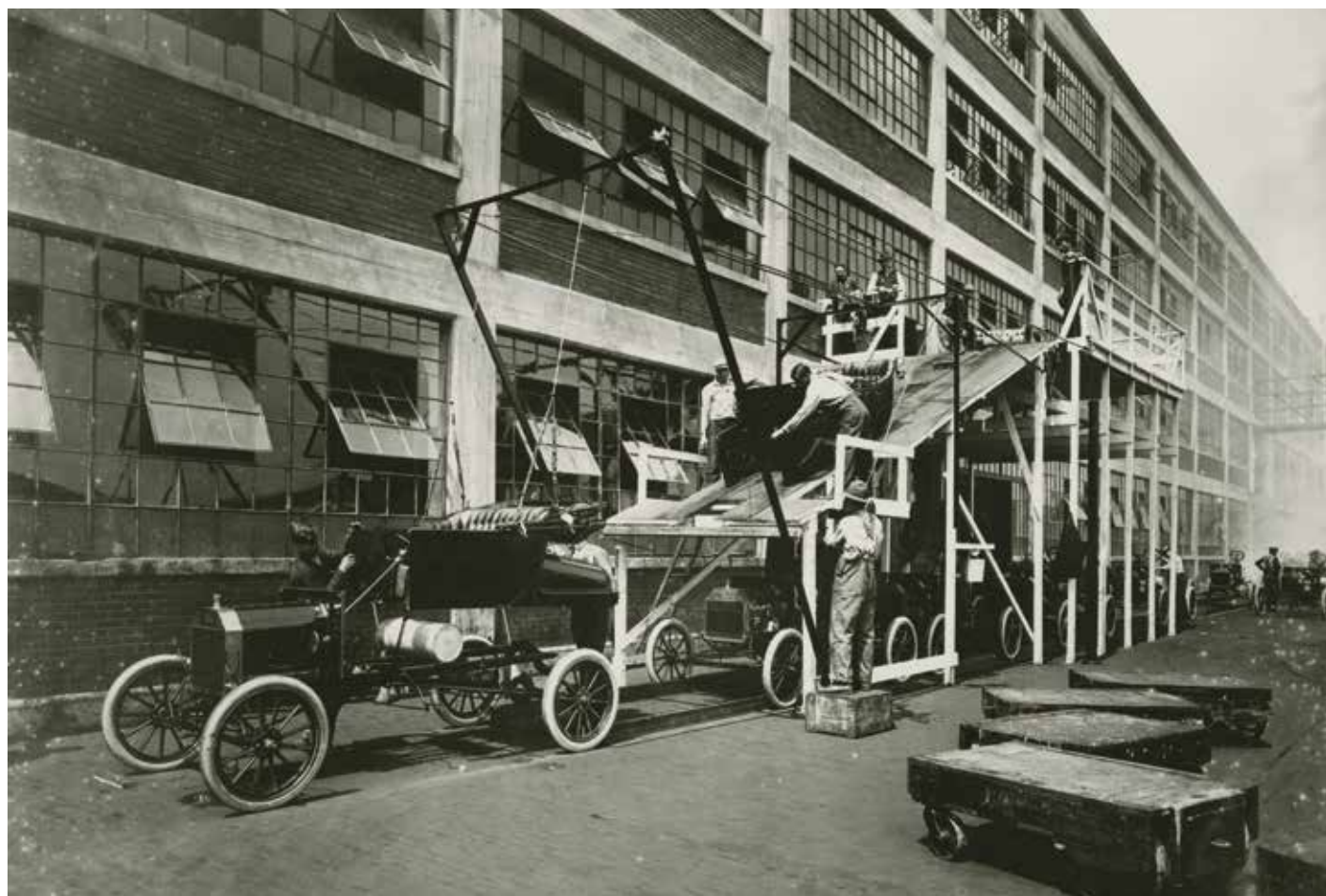
The Model T “body drop,” mating a body and chassis, circa 1914.
