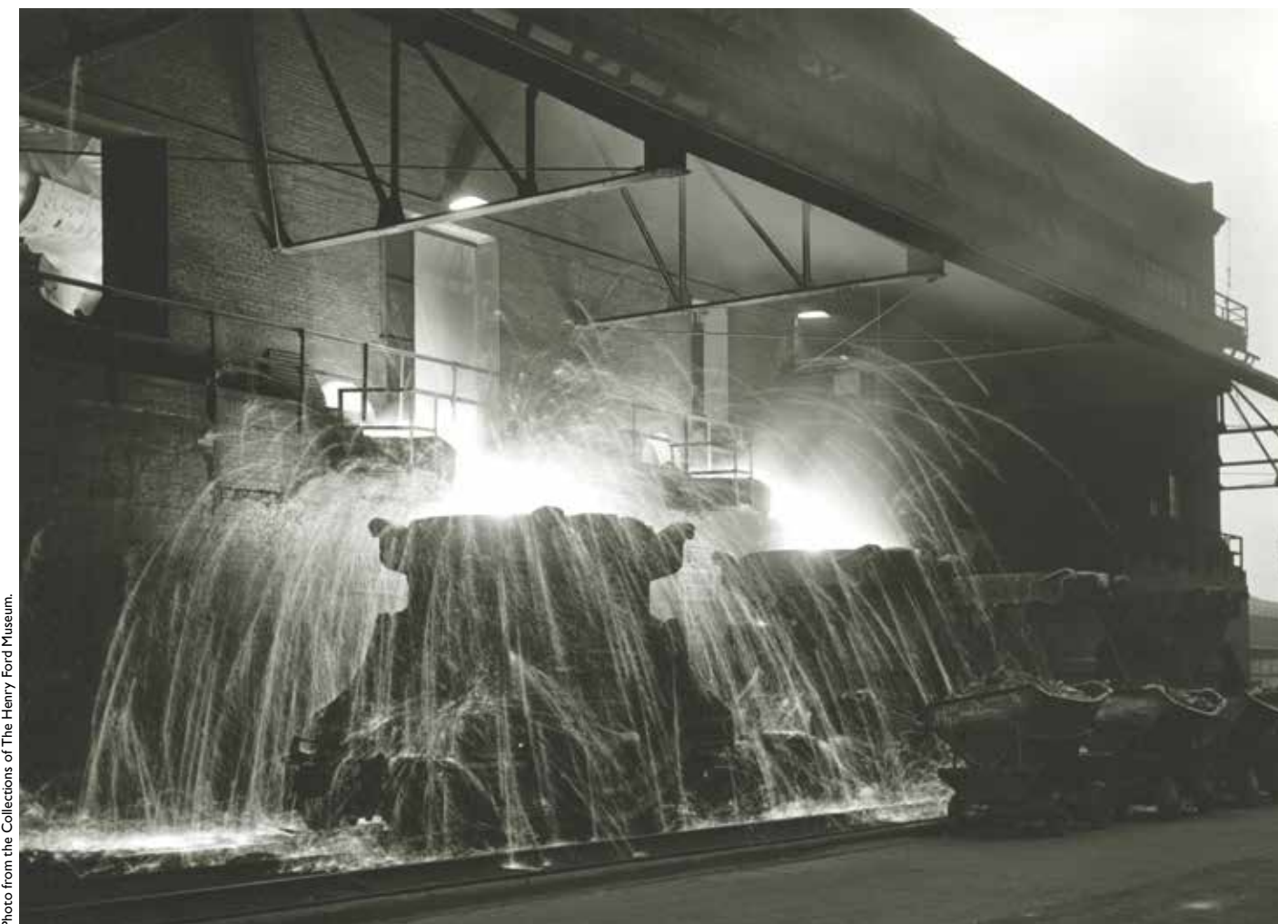
Molten iron pours from a blast furnace at the Rouge in 1932.
