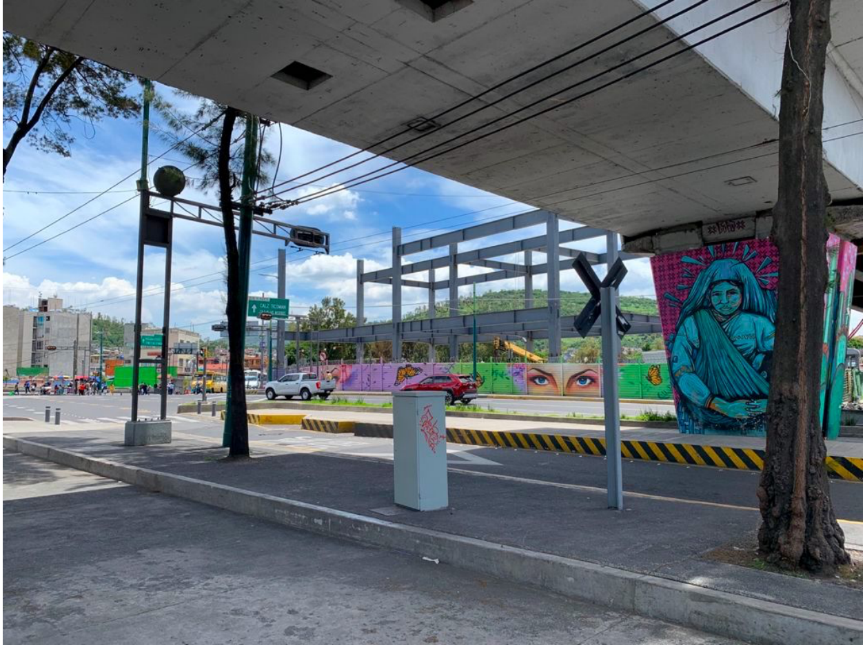
Construction site for a modern transportation hub and commercial mall outside a subway station: a menace for the permanence of street vendors. Photo credit: Irene Farah
