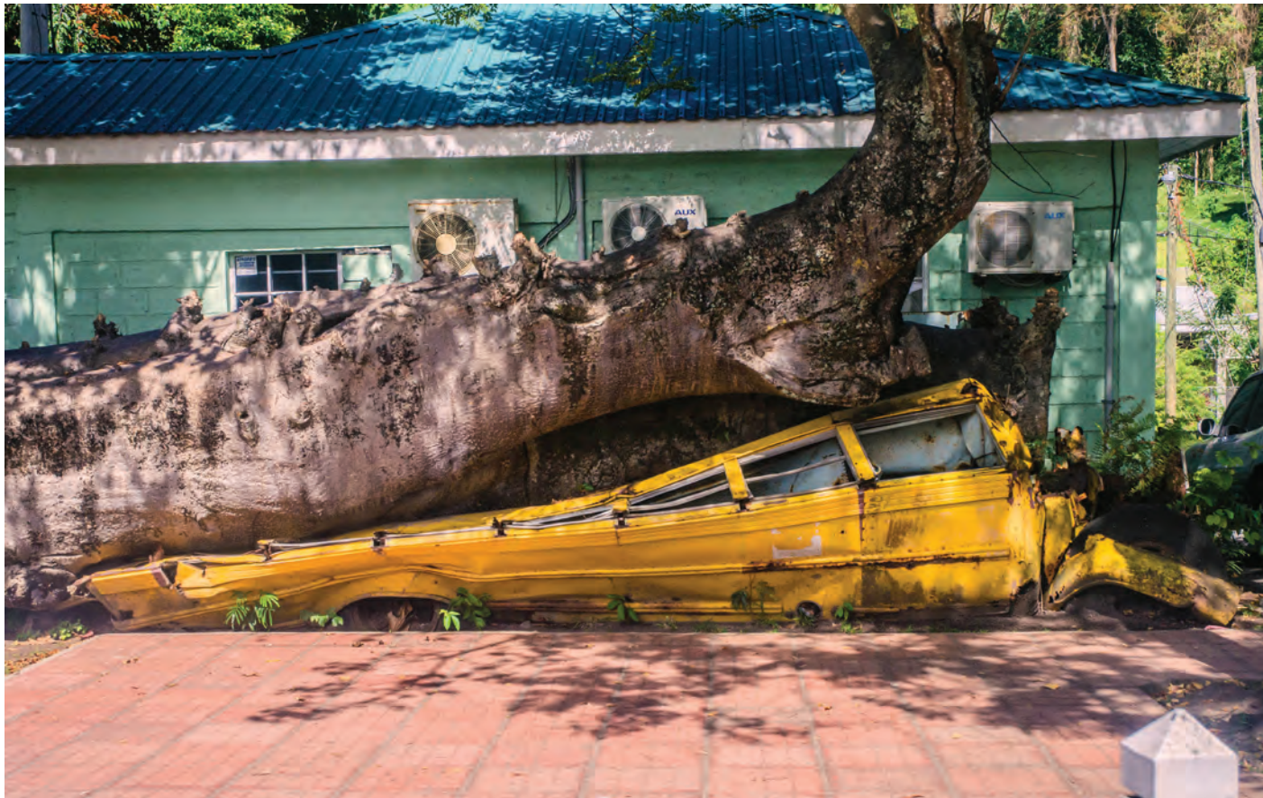
A crushed bus from Hurricane David (1979) remains as a memorial on the island of Dominica.
