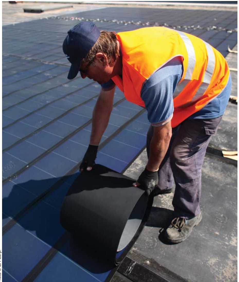
A worker rolls out United Solar Ovonic material on the roof of the General Motors plant in Zaragoza, Spain.
